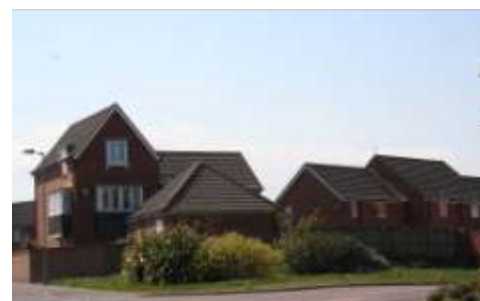
Housing at Grangemoor Farm
